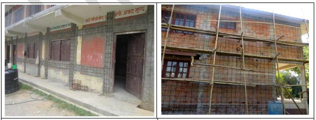
Fig13: Strengthening of infill masonry wall of RC frame building through RC Splint and Bandage method
