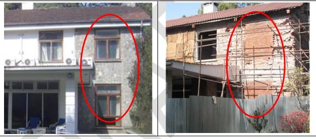
Fig 15: Removal of openings to improve the configuration
