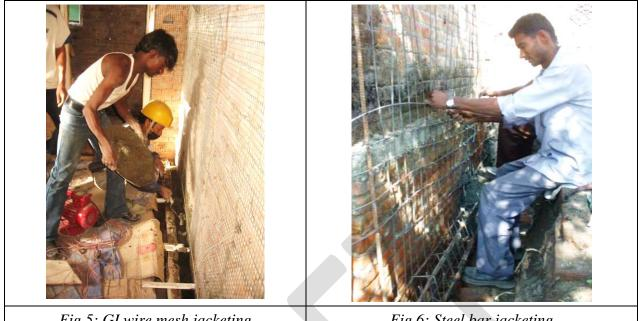
Fig 5: GI wire mesh jacketing
